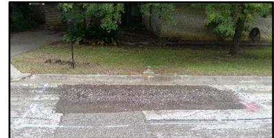
Picture 1: City Utility Backfill Material
