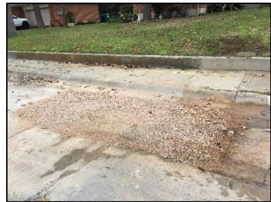
Picture 4: City Utility Backfill Material
